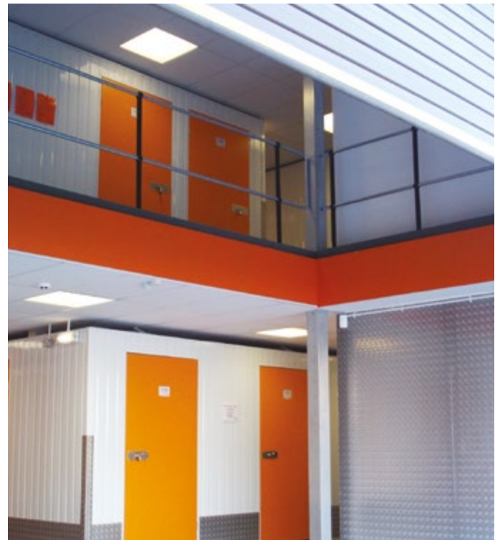
Fire rated mezzanine floor
