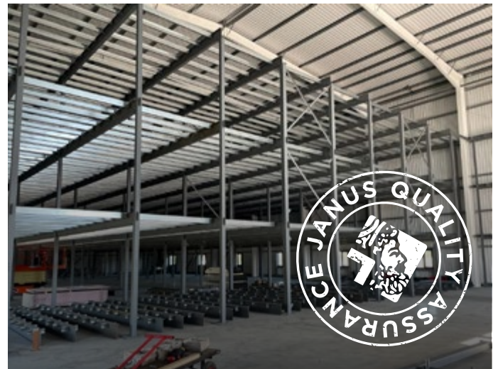
Bare steel mezzanine awaiting installation of decking and fire rating
